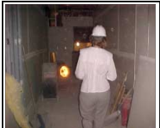
SOLBERG RENOVATIONS —Tracia Hogue cautiously walks in the dangerous cramped basement setting while giving a preview tour of GPRPC's new home... story continued on Page 3.
